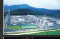
Electro Electric Systems Division
